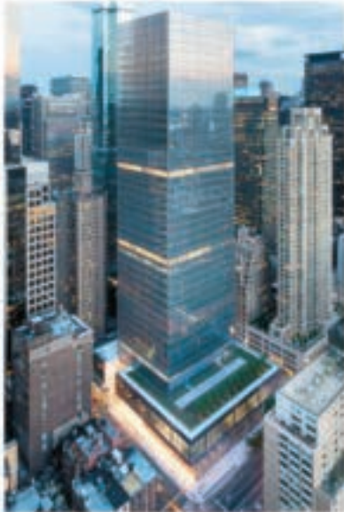
E-J ELECTRIC INSTALLATION CO. LONG ISLAND CITY, NY
